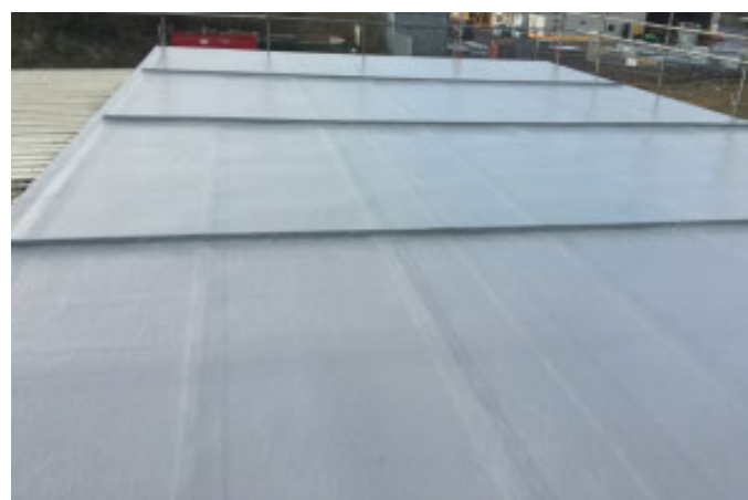
Expose System, Polymarble Laying on Roof Slab
