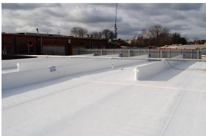
Expose System, Polymarble Laying on Roof Slab
