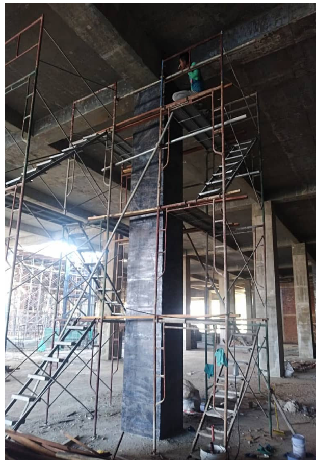
Build Wrap Pro 300 apply on Column
