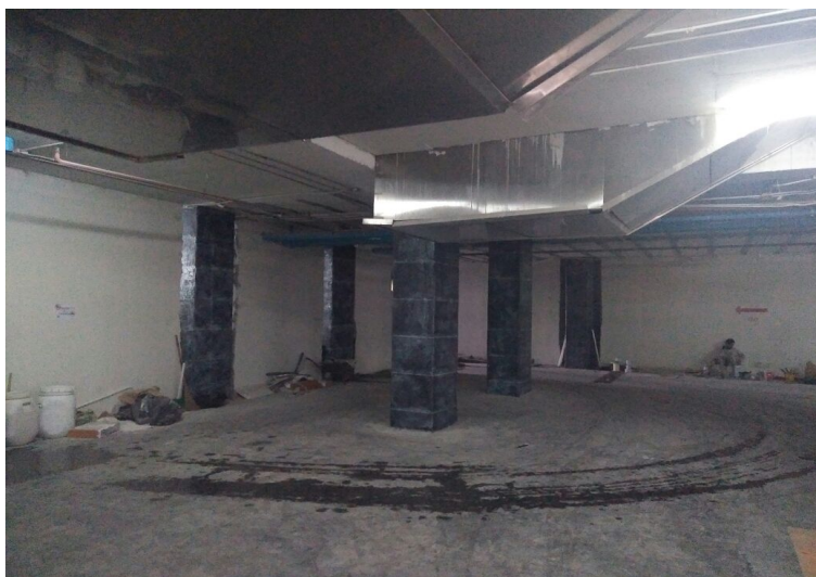
Build Wrap Pro 300, apply on Column
