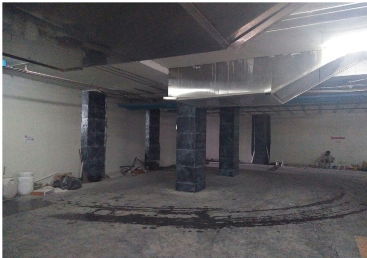
Build Wrap HS 300, apply on Column
