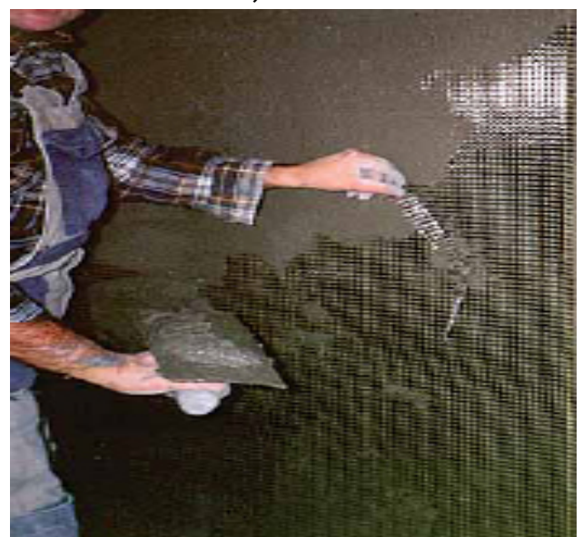
Install on Build Mesh CF 30010 on Wall
