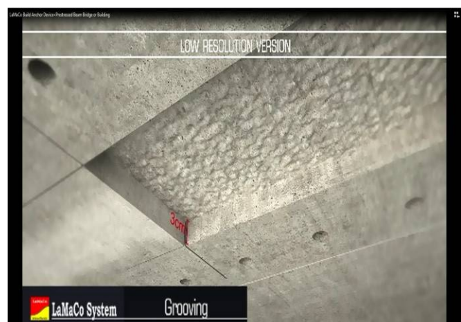
4] Hack Out or Grooving, Depth Set 30mm
