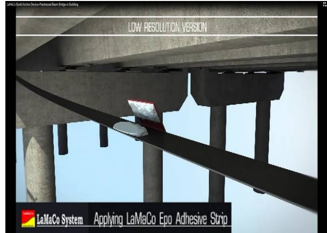
14] Laying the LAMACO-Epo Adhesive Strip
