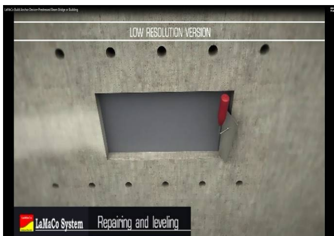
5] Patching to Leveling
